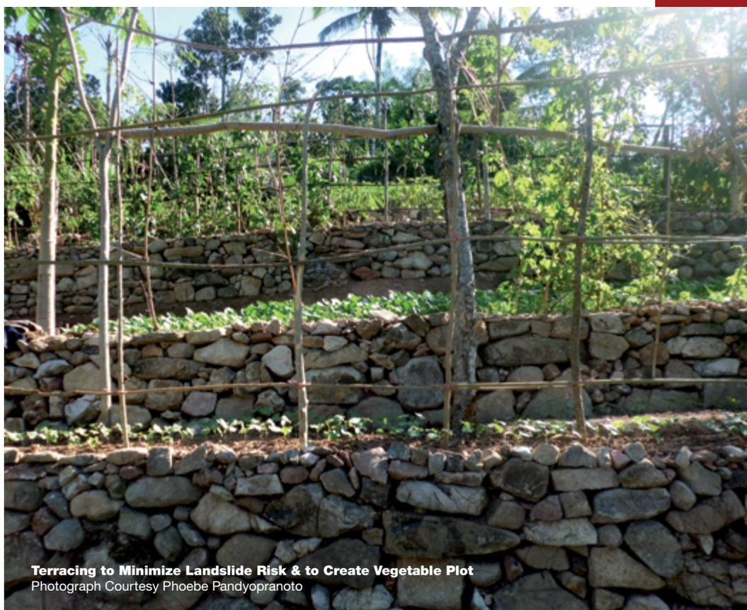
**Terracing to Minimize Landslide Risk & to Create Vegetable Plot**
