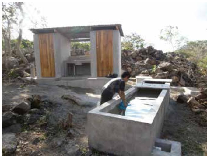
Photo: Bathing and washing facility, built with a water harvesting reservoir, Community of Malpaso
